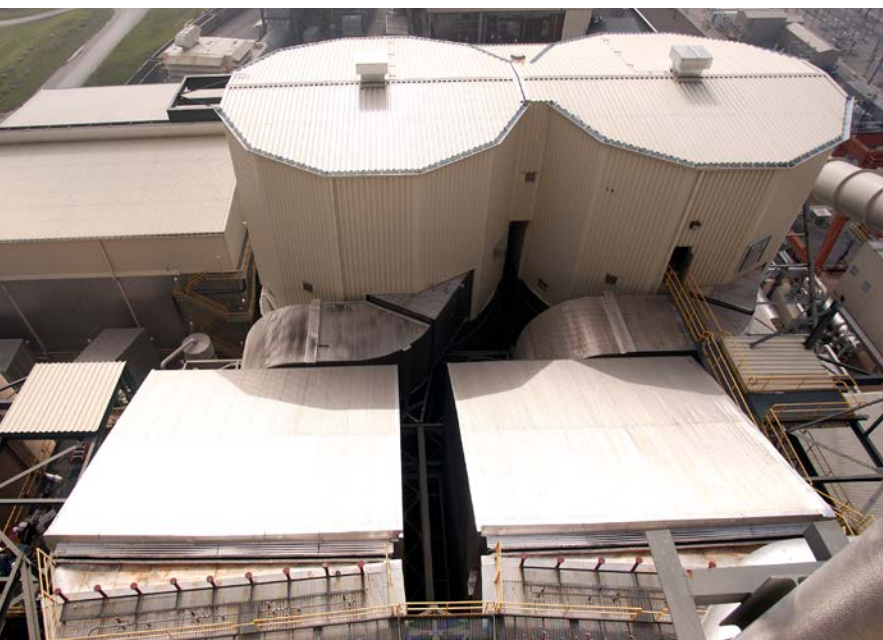
Adjacent SDAs share a common spare atomizer.
