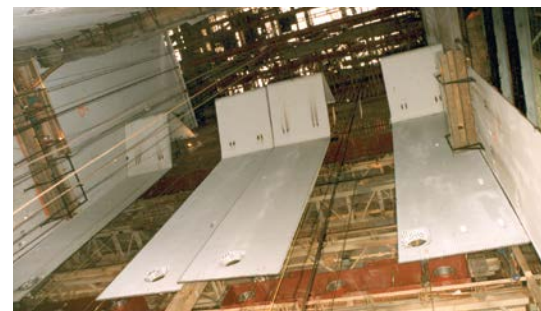
B&W designs its radiant boilers with a large furnace arch to prevent hot gases from bypassing the closely spaced superheater sections. This improves heat transfer and reduces the slagging potential in the superheater, thereby improving availability and reliability.
